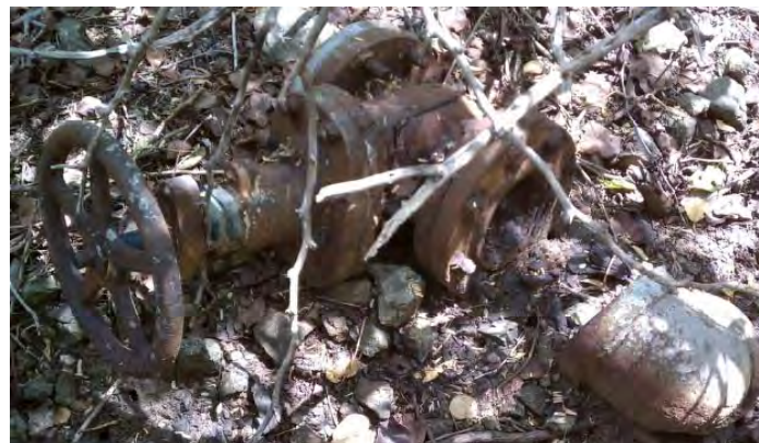
Figure 5: Water Valve in Lower Camp Area
